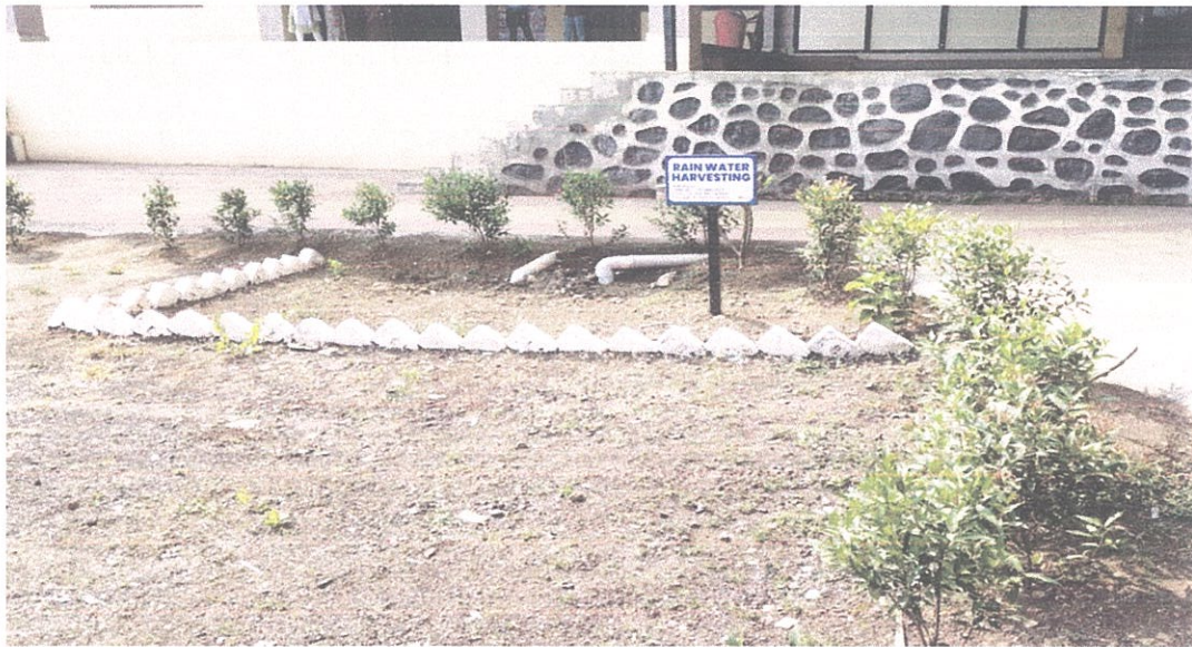
Rain Water Harvesting Plant (side view )
